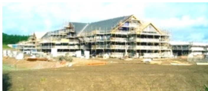
The new Community Hospital takes shape
